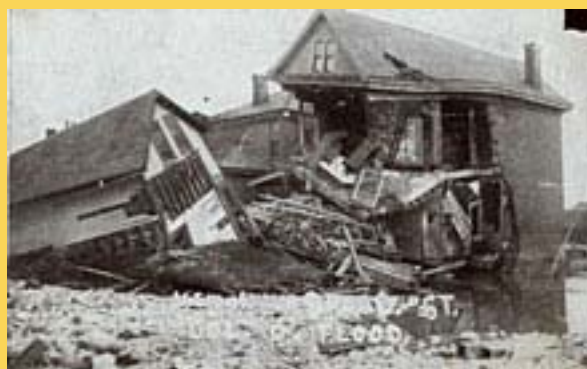
Top: Tornado damage in Omaha, Nebraska, on 23 March 1913. Photo courtesy of the National Oceanic and Atmospheric Administration/Department of Commerce Bottom: Flood damage in Columbus, Ohio. Photo courtesy of Steve Holt/Mitretek Systems
